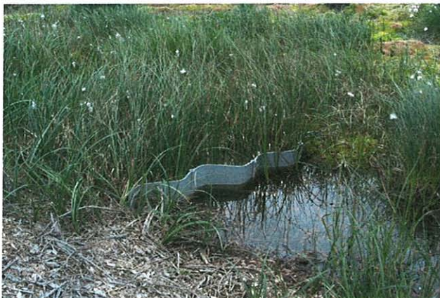
A plastic piling dam on Grain Heads Moss
